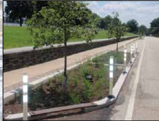
Philadelphia stormwater bumpout Photo Courtesy of: phillywatersheds.org
