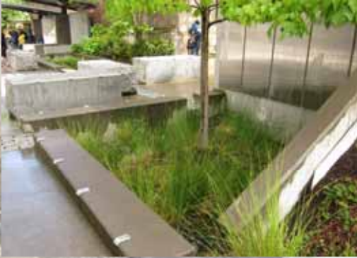
On-site stormwater management Courtesy of: Cory Gallo
