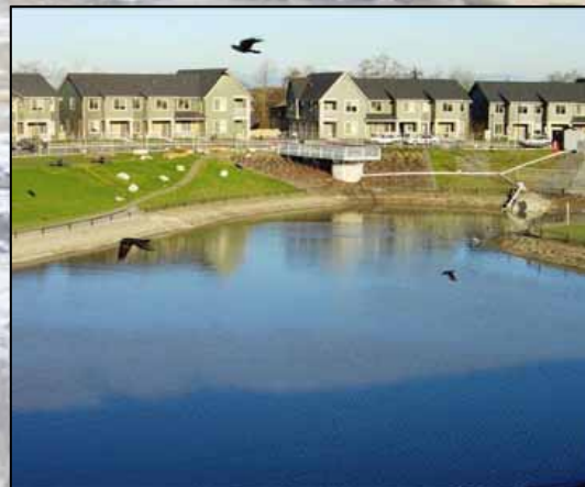
NPDES phase II Stormwater detention pond in Seattle, Washington. Courtesy of: City of Seattle
