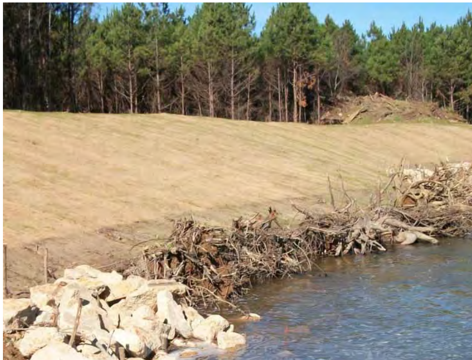
Figure 8. Installed root wads.
