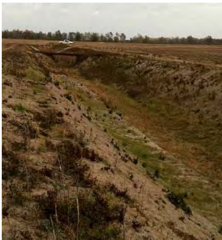
Figure 2. Ditch 2 (Main ditch) following dredging and hydroseeding. A small in-channel floodplain is located \frac{3}{4} of the way down the bank, characteristic of a 2-stage ditch.
