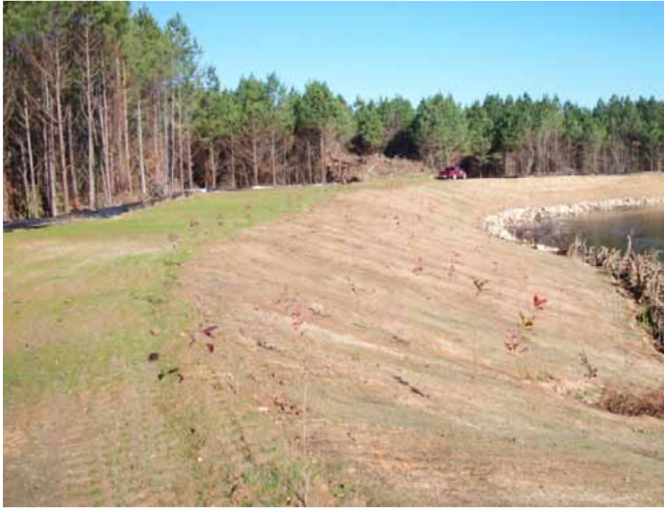
Figure 13 . Post-construction site looking downstream.
