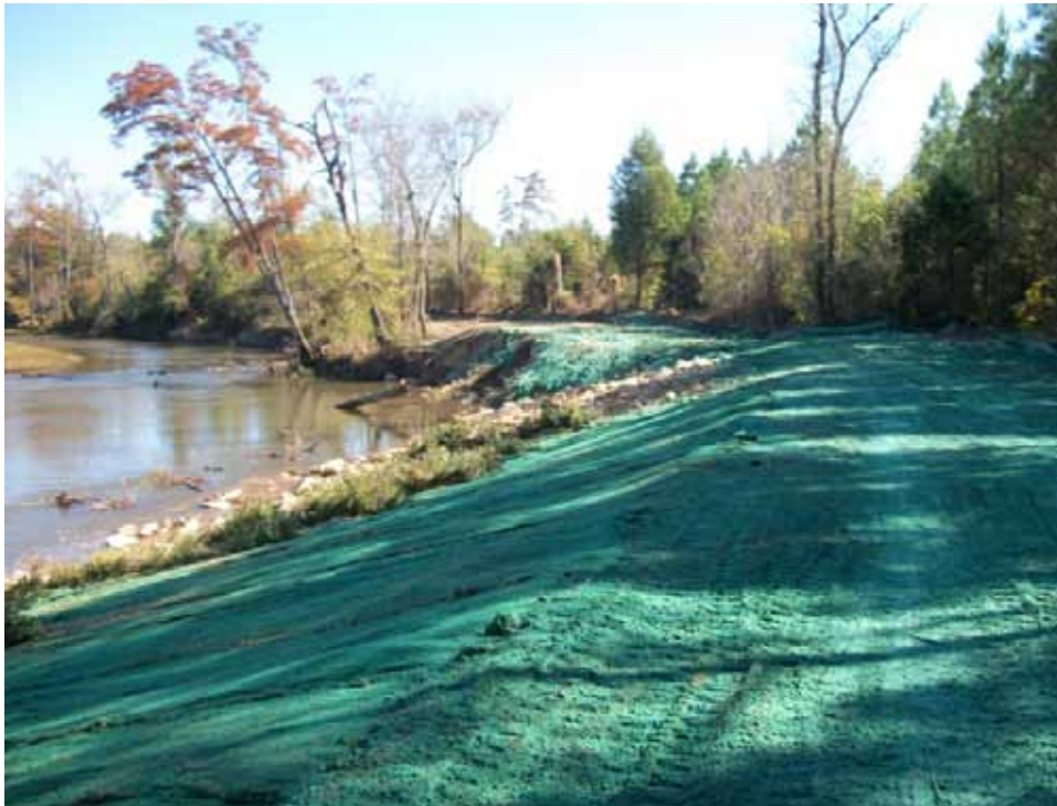
Figure 12. Post-construction site looking upstream.
