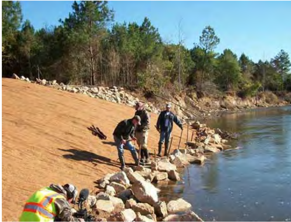
Figure 9. Placement of willow stakes.
