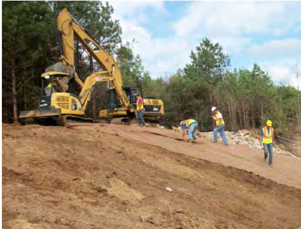
Figure 5. Installation of erosion control blanket.
