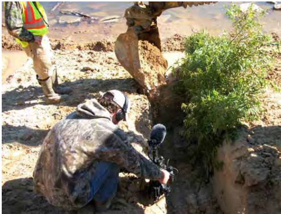
Figure 10. Installation of willow trenches.
