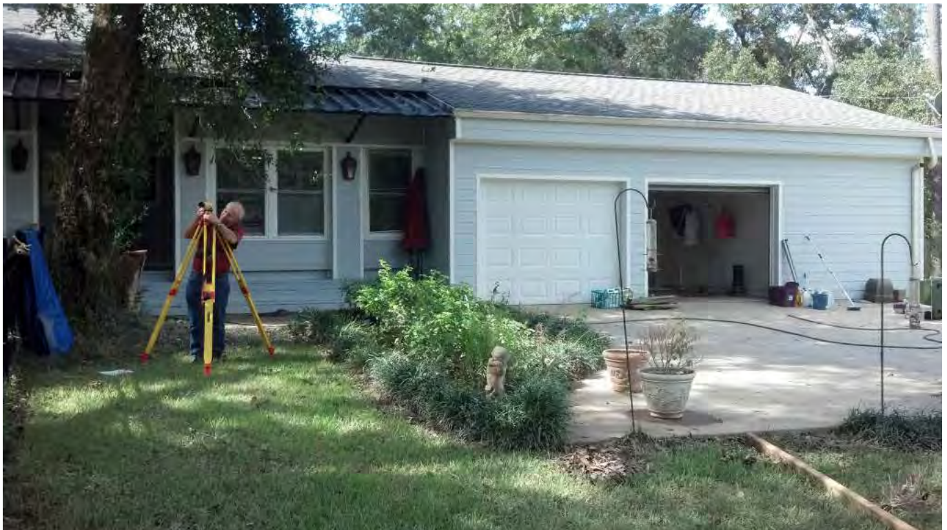
Figure 8. This home on Magnolia Dr. had a clear high water mark inside of the attached garage. Flood survey team members Marty Pope (pictured) and W. Scott Lincoln used this high water mark to help estimate the crest for the Wolf River at Bells Ferry Rd. (GLFM6) forecast point.
