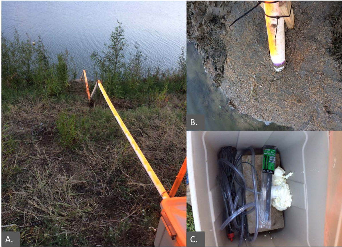
Figure 4. Actual piezometer placed in TWR/OFS placed in System 1. Image A shows PVC pipe housing pressure gauge wiring and sample tubing along bank from the piezometer; Image B shows the PVC pipe where it connects to the piezometer and enters the sediment in System 1; Image C shows wiring and tubing housed in plastic bin on top of the TWR/OFS bank for accessible data downloading.
