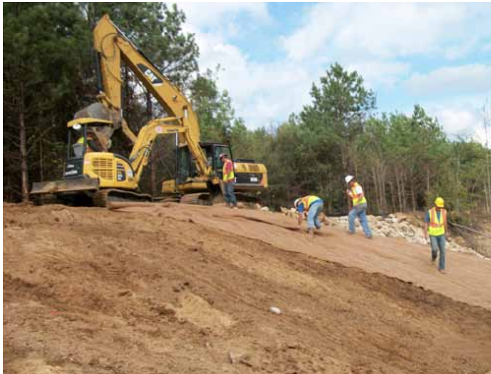
Figure 5. Installation of erosion control blanket.
