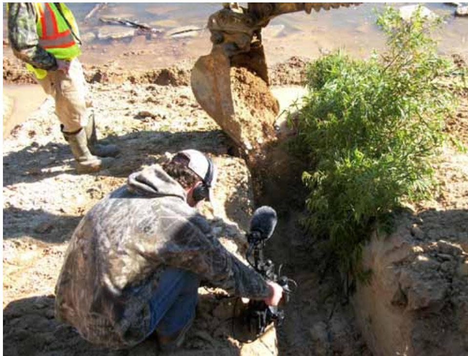
Figure 10. Installation of willow trenches.
