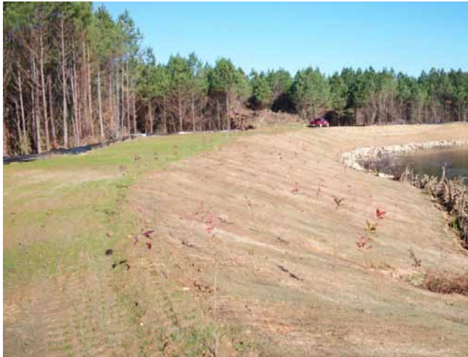
Figure 13 . Post-construction site looking downstream.
