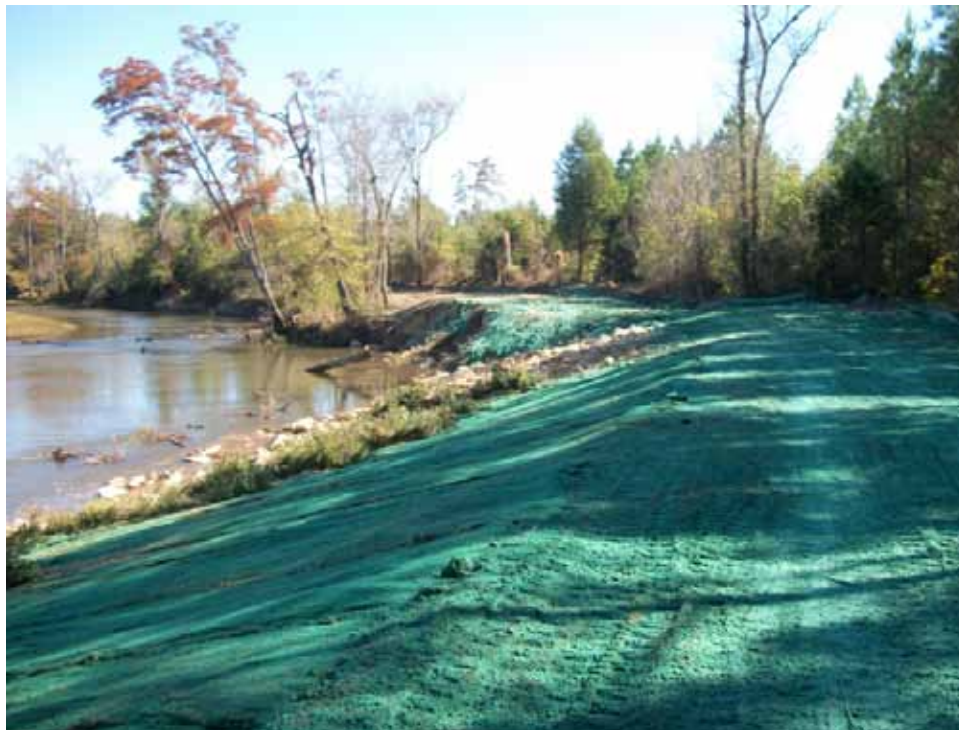
Figure 12. Post-construction site looking upstream.
