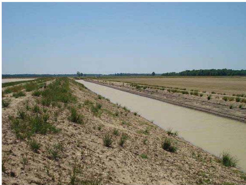
Figure 12: North to south view of a catchment ditch with reservoir on the left and leveled field on the right (Photo: R. Thornton)
